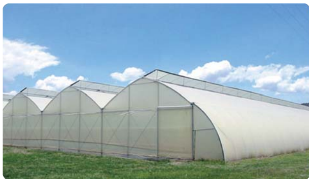
Fig. 7.4 Typical naturally ventilated polyhouse (NVPH)
