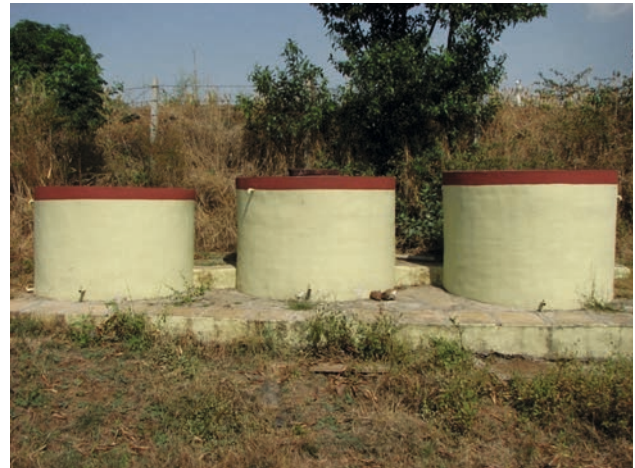
Rainwater harvesting tanks
